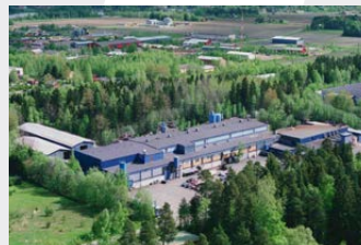
PEIRON OY STEEL FOUNDRY KOKEMÄKI, FINLAND
