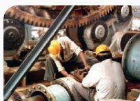
5. On-site supervising and repairs work
